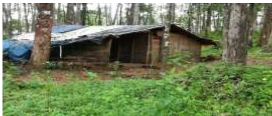
Fig.3. present house condition.
